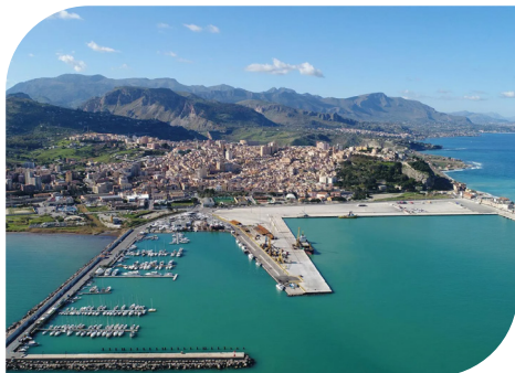
Transport & Infrastructure Porto di Termini Imerese Integrated Security Management
